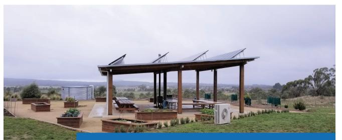
This is an example of a larger outdoor structure – not quite a "shed" but with sufficient shading as to be usable most of the year. Notice the photovoltaic arrays on the roof of the structure. These can be used to power project work within the enclosure itself or be connected to the school's central power supply. Ballarat Grammar School, Victoria, Australia. Photo: Roni Zimmer Doctori
